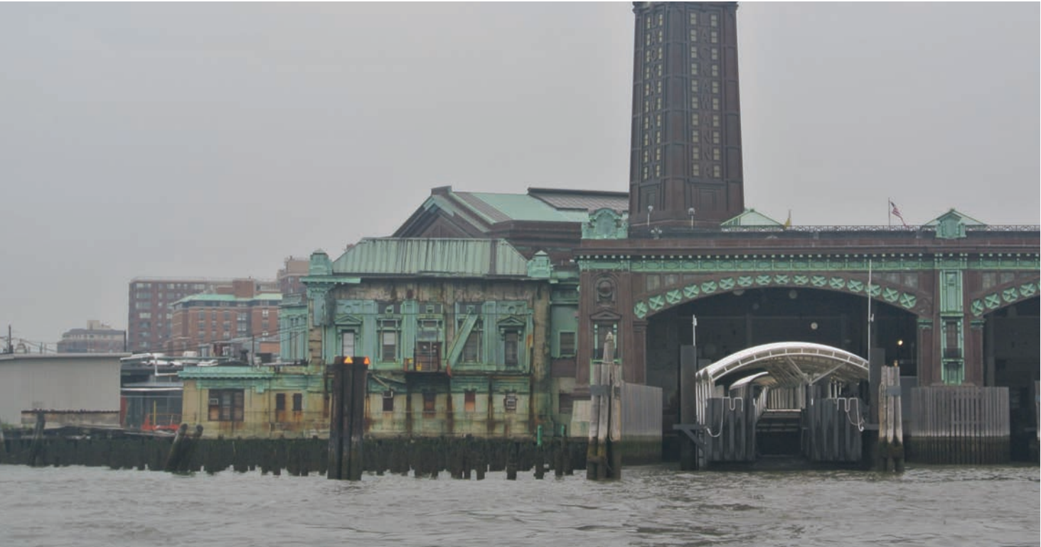
Photograph 3.2 Hoboken Terminal, wood-crib bulkhead
