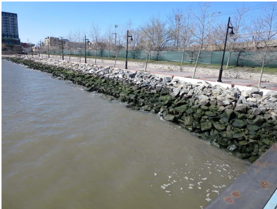
Plate 14: Riprack and Wood Bulkhead to East of Weehawken Cove within Northern Segment of Alternative 1. View Southwest. (TF 4/5/2016).
