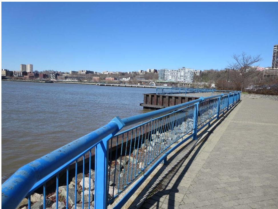
Plate 16: Cobblestone Paths and Riprack Bulkhead Enforced with Iron Bulkhead along Shoreline of Weehawken Segment of Alternative 1. View Southwest. (TF 4/5/2016).
