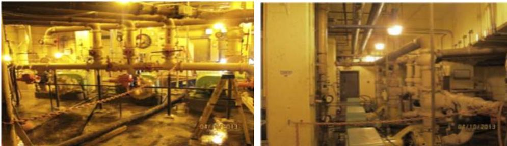
Secondary sludge is pumped from the clarifiers to a sludge storage tank prior to sludge thickening. The sludge pumping system includes three (3) Wemco vortex type sludge pumps.
