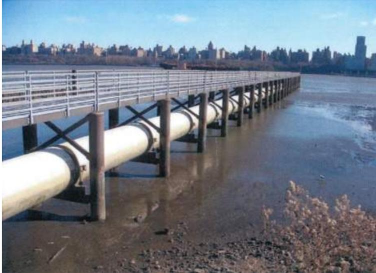
The River Road outfall pipe was inspected by divers in May 2010. It was determined that the pipeline and supporting structure are in fair condition overall, with a few repairs required to remedy some deflection in the pipeline as well as typical maintenance on minor cracking and coating loss on the support structure. There are no current capital improvement projects in progress for the River Road Outfall, and there are no future proposed capital improvement projects.
