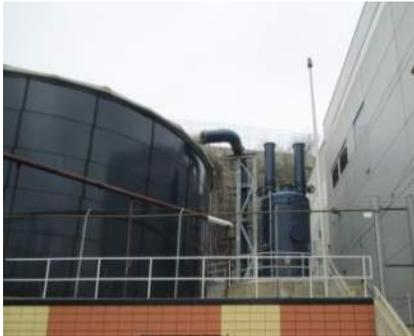
The influent and effluent gates need replacement and new air monitoring equipment in the building is needed to detect Hydrogen Sulfide (H<sub>2</sub>S), Lower Explosive Limit (LEL), Carbon Monoxide (CO) and Oxygen (O<sub>2</sub>). The current unit monitors LEL only.
