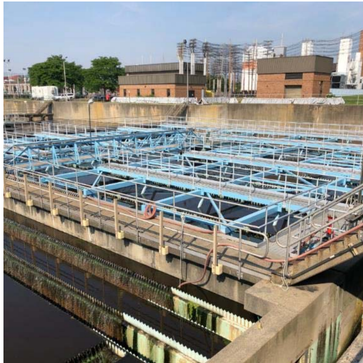
Figure 4-23: Effluent Launder in Bay C, FC 1
