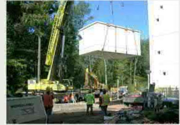
Verona Gebhardt Pumping Station – precast concrete structure
