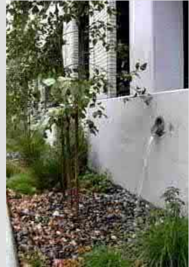
Water from the roof flows from this disconnected downspout into the ground through a filter of pebbles.
