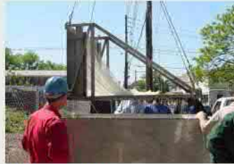
Solids/Floatables Control Facilities – netting frame being lowered
