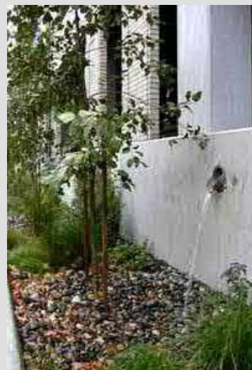
Water from the roof flows from this disconnected downspout into the ground through a filter of pebbles.
