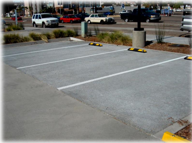
Figure 4-6 - Pervious Concrete Panel
