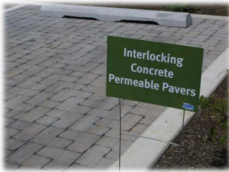
Figure 4-7 - Permeable Interlocking Concrete Pavers
