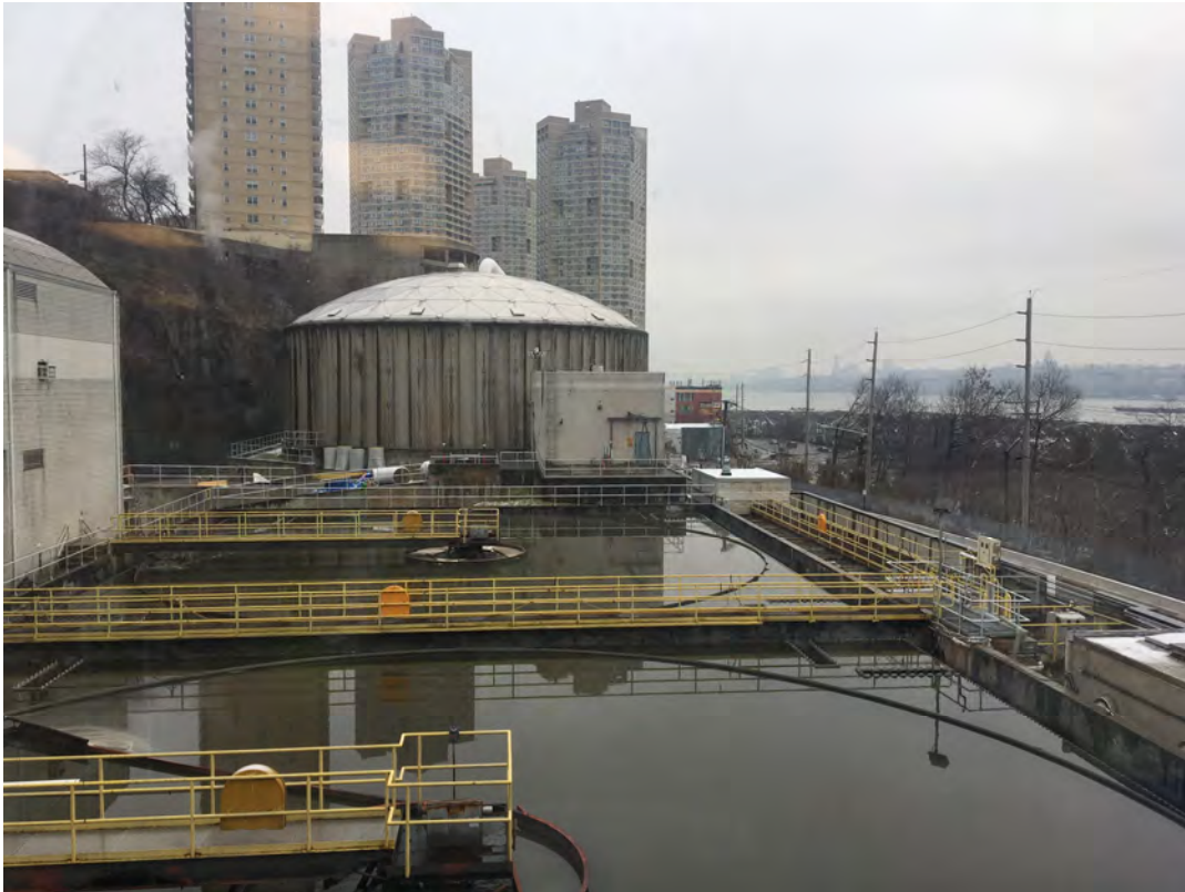
Figure 6-8. Secondary Clarifiers and Chlorine Contact Tank
