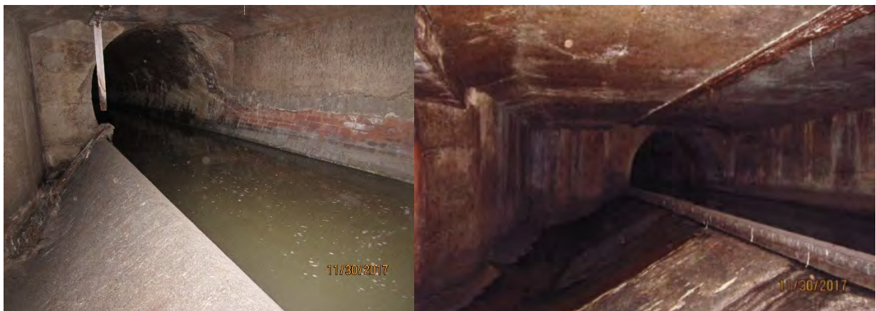
Figure 3-9. Existing Side-Flow Weirs
