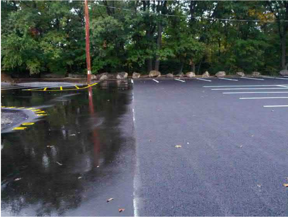
Figure 4-5 - Porous Asphalt Parking Lot
