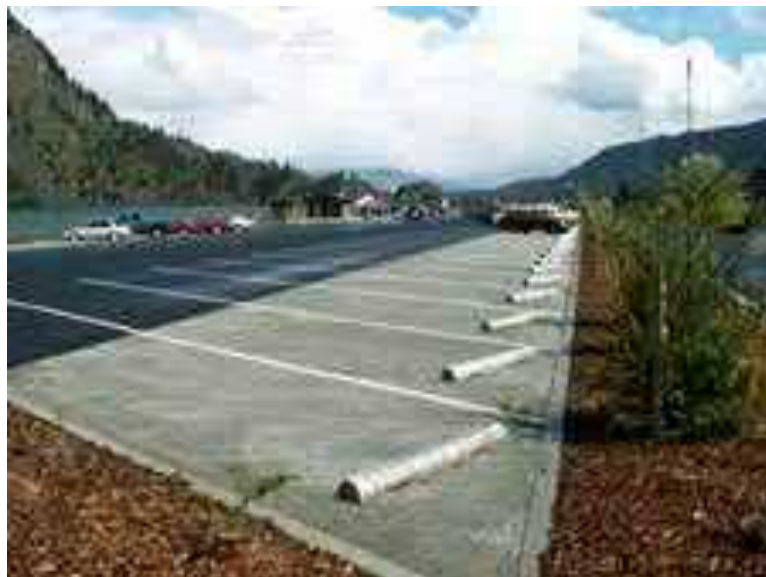
Figure 4-6 – Pervious Concrete Panels
