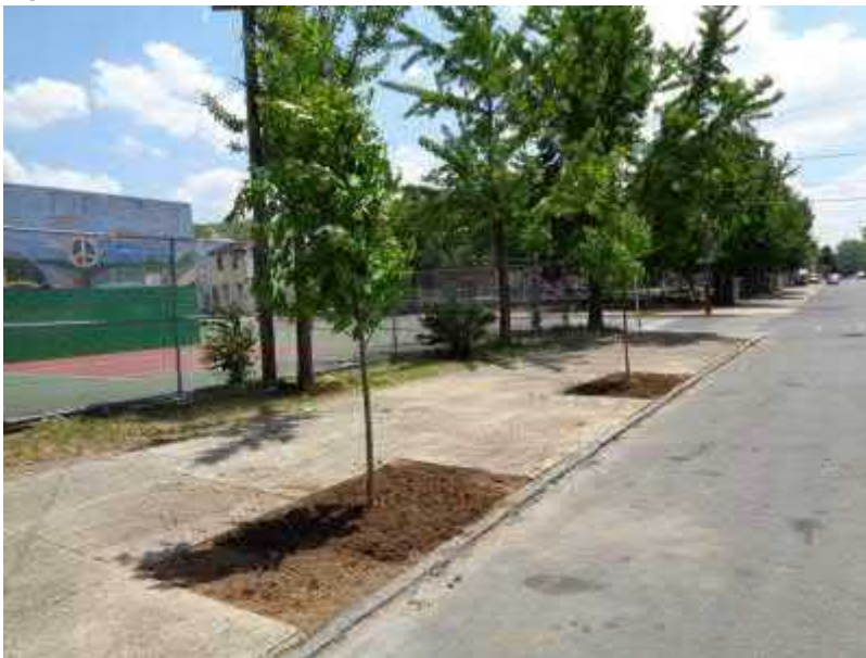
Figure 4-3 - Photo of Enhanced Tree Pits
