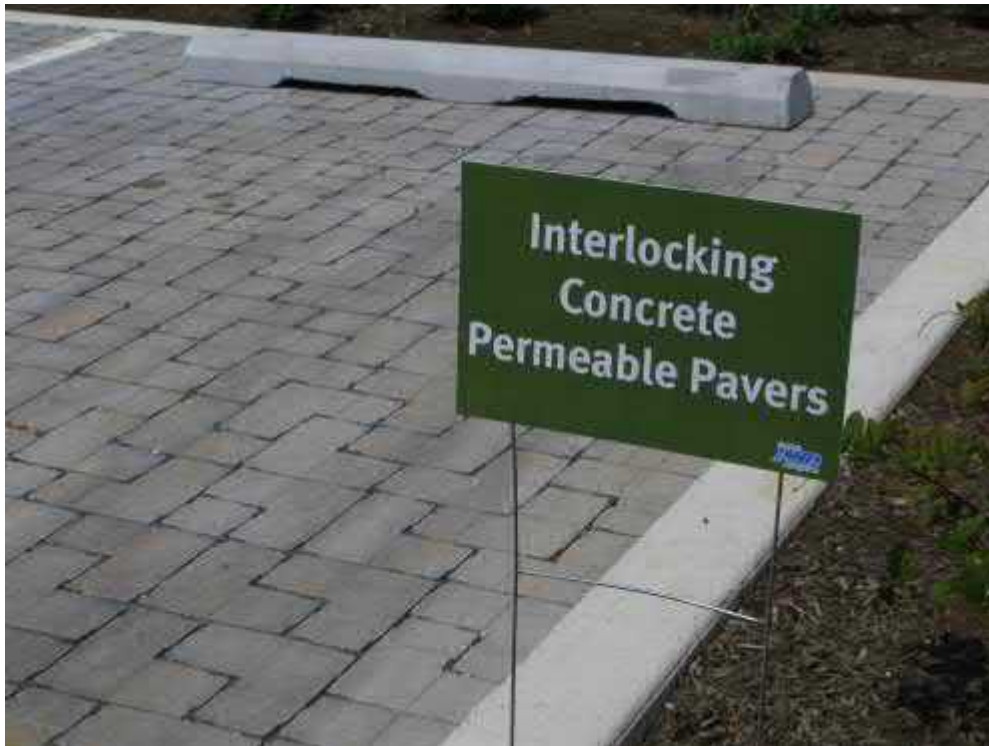
Figure 4-7 – Permeable Interlocking Concrete Pavers (source: EPA)
