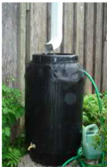
Figure 5-2 Rain Barrels
