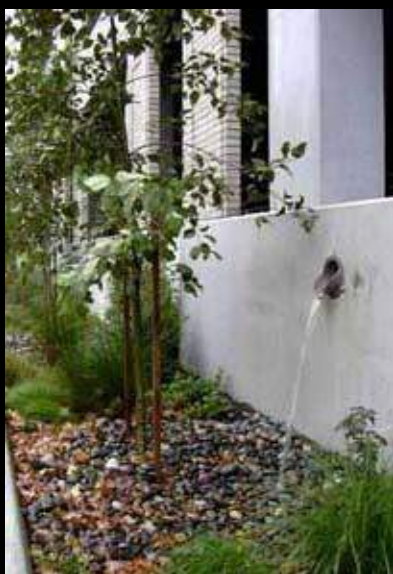
Downspout Disconnection
