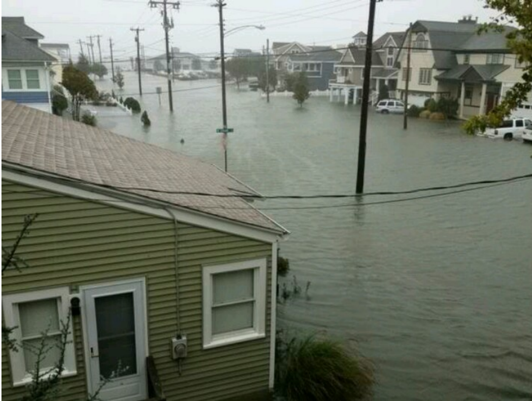
Flooding in NJ shore towns- Hurricane Sandy
