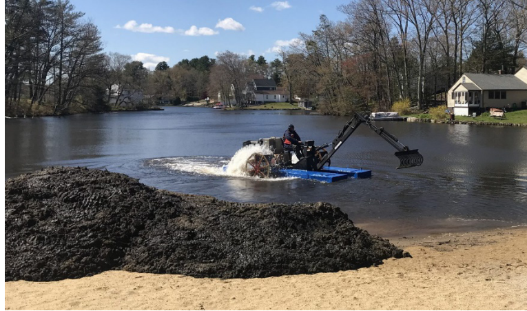
Figure 1. A hydroraking vessel in the water. Material hydroraked is seen on the shoreline in the foreground. Image from Solitude Lake Management.
