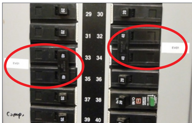
Figure 11. Level 2 Charging Station 240-volt (40 amp) circuits breakers and examples of empty breaker slots Courtesy Energetics Incorporated
