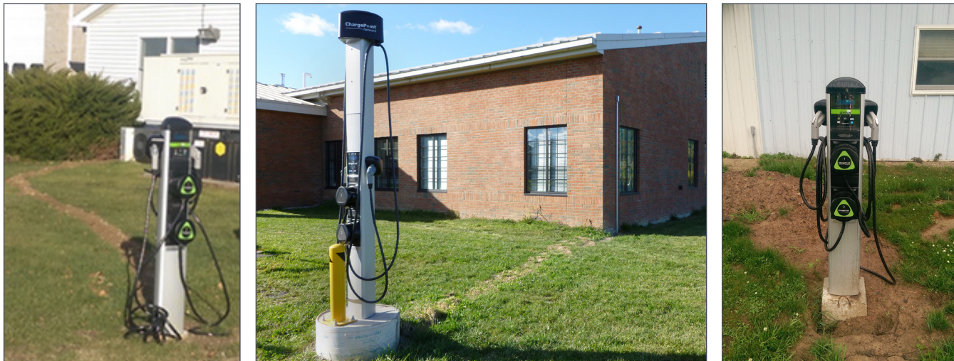
Figure 14. Charging stations can be installed by cutting and repairing (left and center photos) and tunneling under (right) concrete walkways Courtesy Energetics Incorporated
