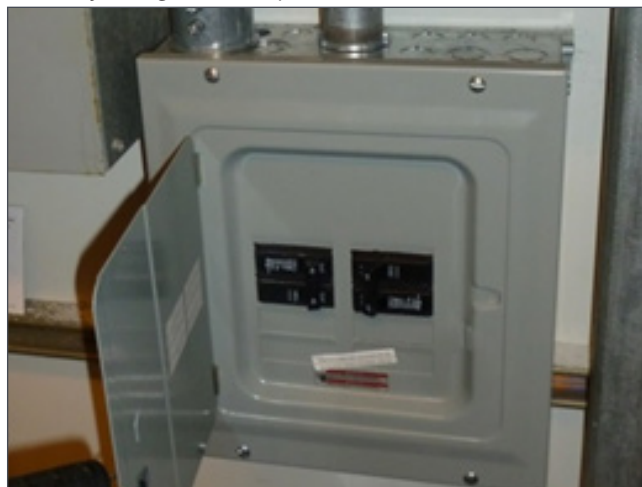
Figure 12. Charging station circuits may require an added subpanel, such as this one, if space in the main panel is limited
