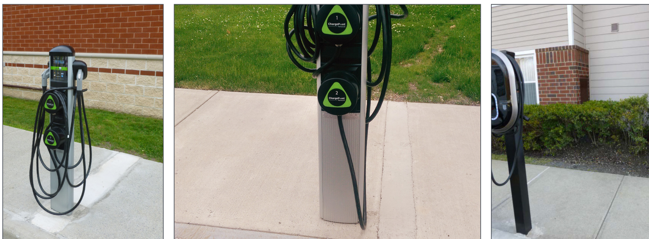
Figure 15. Installing charging stations in parking lots usually requires either cutting and repairing (left and center) and tunneling under (right) pavement Courtesy Energetics Incorporated
