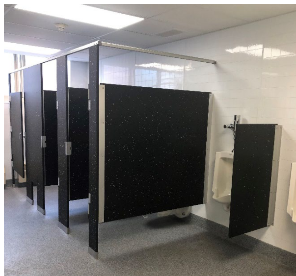
Lower Cape May Regional High School restroom with newly installed high efficiency WaterSense toilets and urinals.
