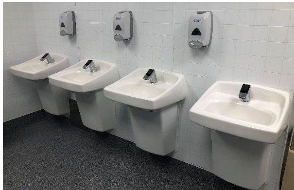
Lower Cape May Regional High School restroom with newly installed high efficiency WaterSense sinks.
