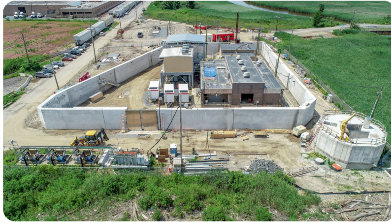
Middlesex County Utilities Authority's Sayreville Pump Station with a flood wall constructed around the facility.
