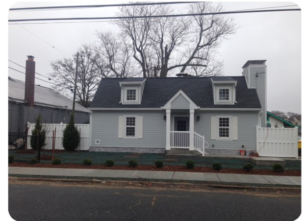
South Monmouth Regional Sewerage Authority's Lake Como Pump Station. This pump station was built outside of the flood zone and was built to look like a residential house to blend into the neighborhood.
