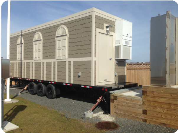
South Monmouth Regional Sewerage Authority's Pitney Mobile Pump Station. This pump station can be moved during storm or flooding events.
