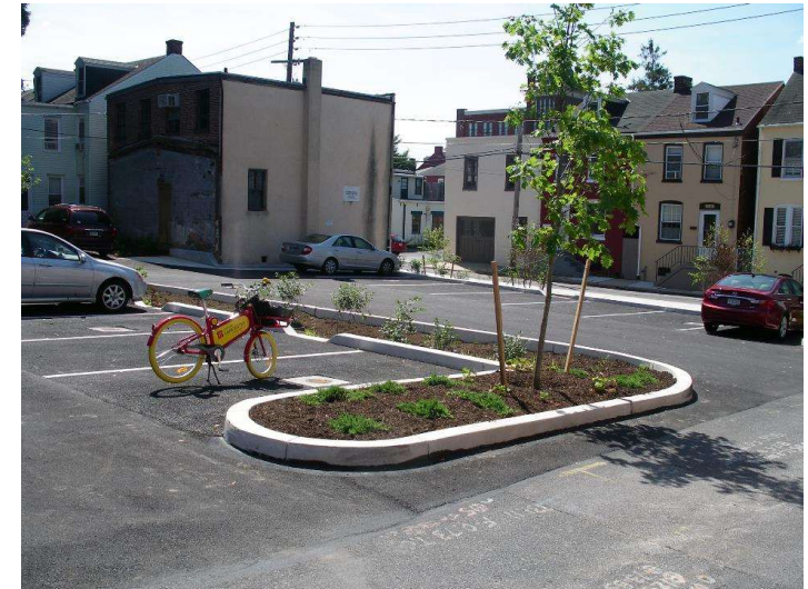
Grant funded porous asphalt and bioretention rain garden in Church parking lot.
