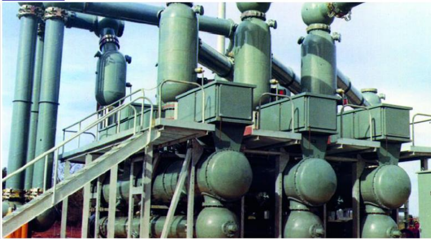
The world's first 800 kV GIS - Joshua Falls, VA – 1980 - DELL ALSTHOM
