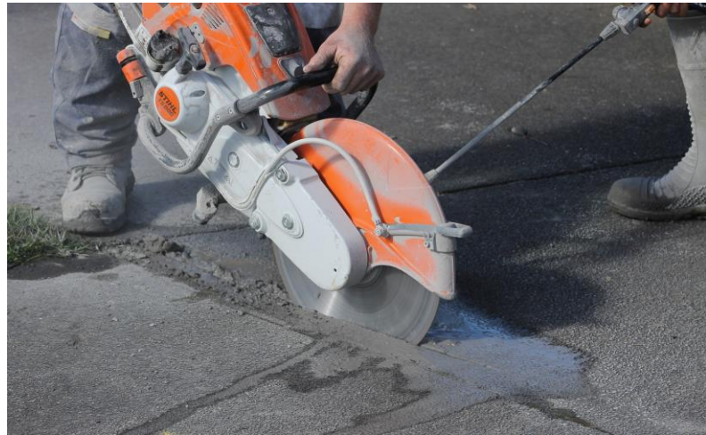
Wet cutting methods
