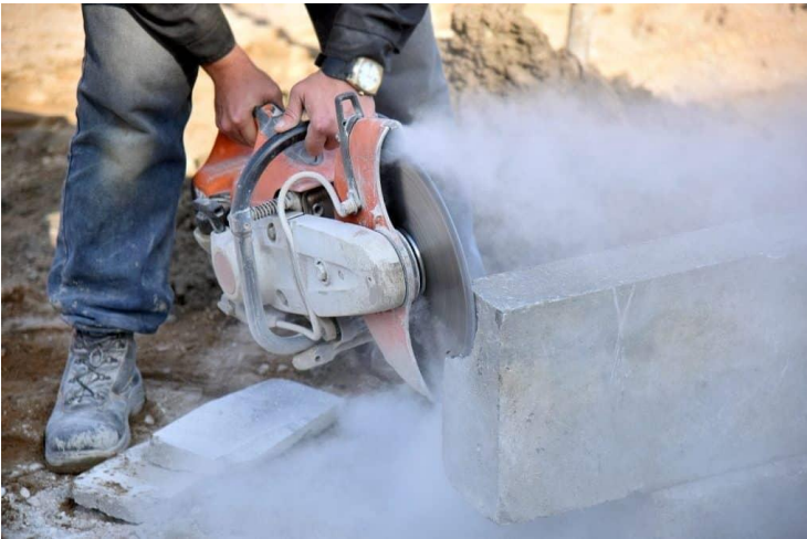
Circular saw cutting concrete with no controls
