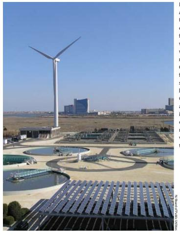
New Jersey's **Atlantic County Utilities Authority** commissioned a five-turbine, 7.5 MW wind farm at its wastewater treatment plant in Atlantic Citv in 2005. Also featuring a 500 kW solar PV array, it became Atlantic City's most unlikely attraction during its first year of operation, when more than 4,000 visitors toured the site.
