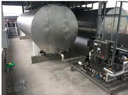
Reagent Bulk Tank
