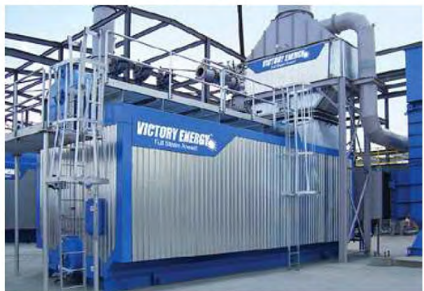
VOYAGER® O-type boiler with EXPLORER® economizer installed.
