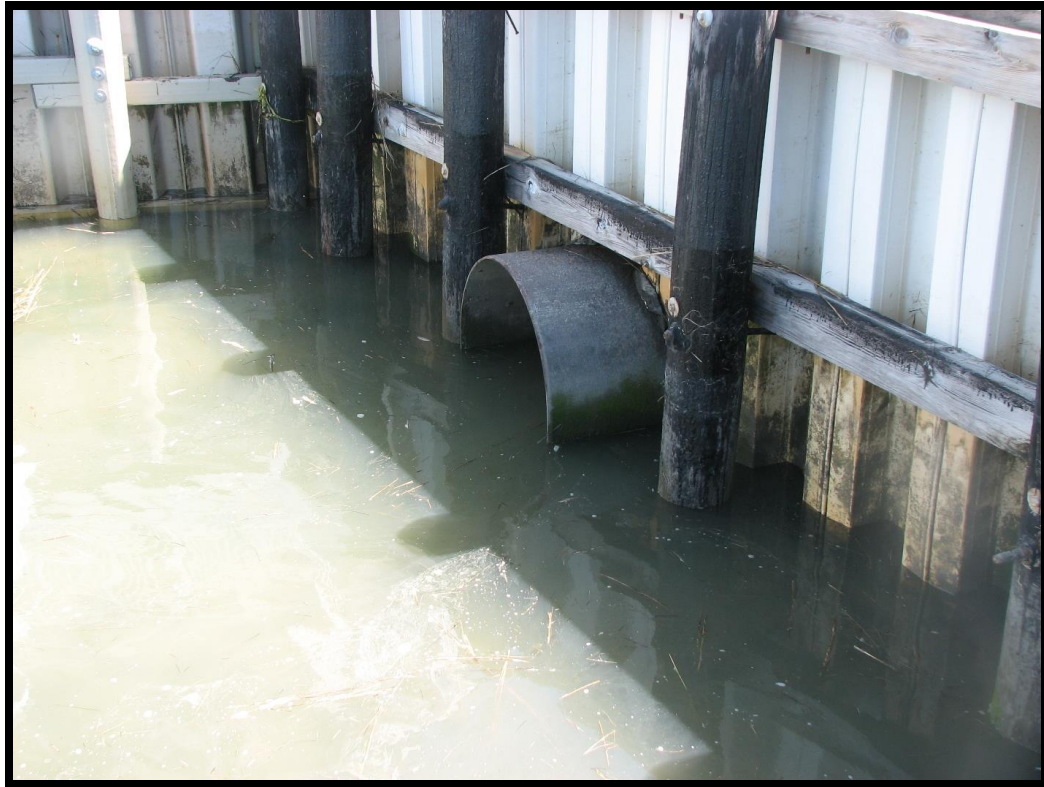
FIGURE 21: STORMWATER OUTFALL PIPE EXTENDING TOWARDS LUDLAM THOROFARE AT THE WEST END OF 58 TH STREET IN SEA ISLE CITY.
