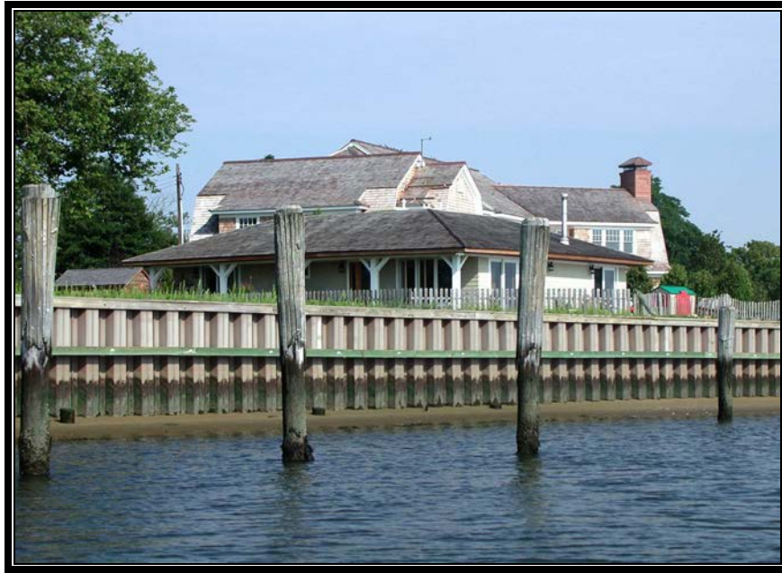
FIGURE 7: NEW BULKHEADING, THE WOODEN POLES ARE REMNANTS OF THE OLD BULKHEAD
