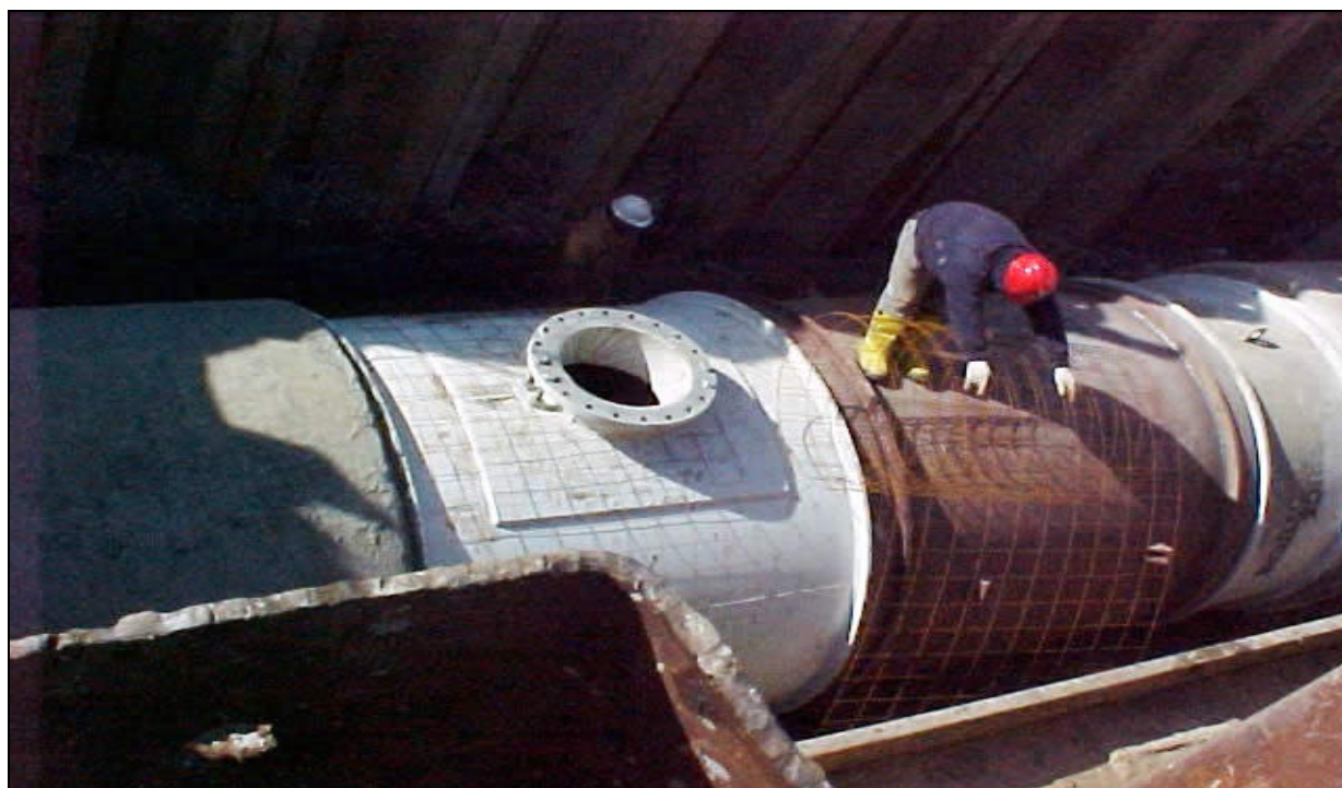
FIGURE 19: MCUA 102 SAYREVILLE RELIEF FORCE MAIN REPAIR (SOURCE: MCUA)
