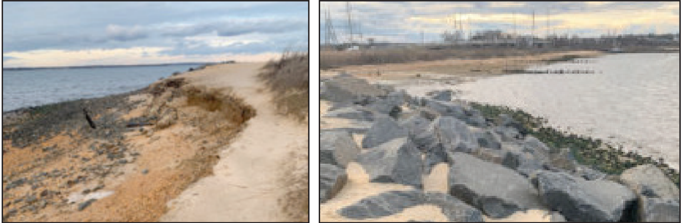
Beach erosion and revetment wall at Paul's Beach. (NJ Flood Mapper, 2017)
