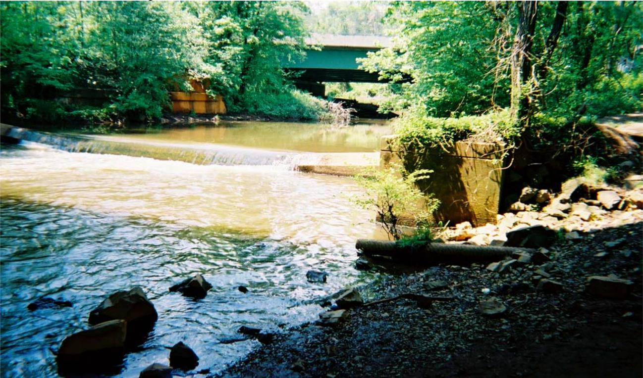
Run-off to Manasquan River at USGS Station 01408000 (Manasquan River at Squankum). Unconsolidated soil covers an unprotected slope and is washed down by runoff to a pool formed by a Squankum dam. The water quality sampling site 01408000 is approximately 60 feet from this site.
