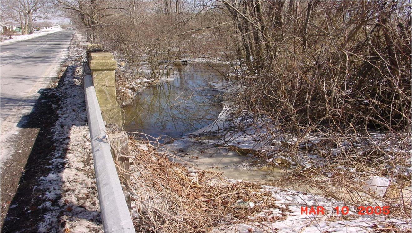
Long Brook at Howell. Fine sand and silty material is deposited into the stream bed by the runoff water. Silty deposit fills approximately  $\frac{3}{4}$  of the total channel width.
