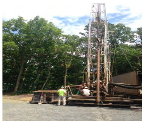
Drilling of a Drinking Water Well at the Berkeley Twp. MUA
