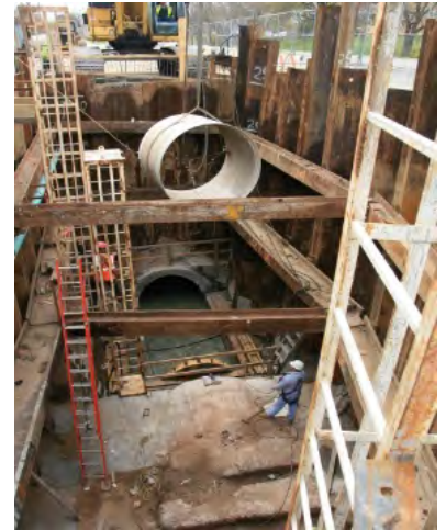
Passaic Valley Sewerage Commission Interceptor Slip Lining
