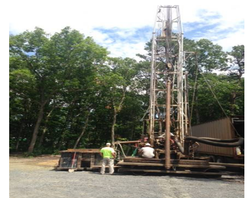
Drilling of a Drinking Water Well at the Berkeley Twp. MUA
