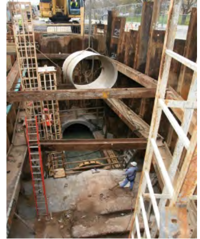
Passaic Valley Sewerage Commission Interceptor Slip Lining
