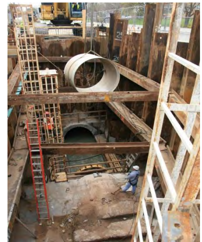
Passaic Valley Sewerage Commission Interceptor Slip Lining
