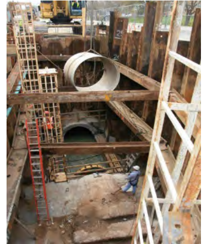
Passaic Valley Sewerage Commission Interceptor Slip Lining
