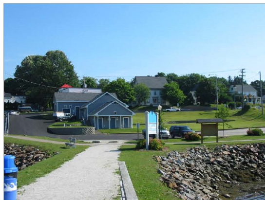
Bucksport CSO Facility From Fishing Pier
