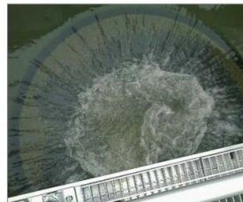
The low maintenance Swirl-Cleanse screen is self-cleansing with no power requirement
