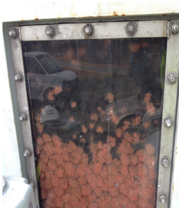
Figure 7.8 CSO solids on FlexFilter media
