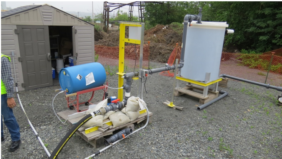
Figure 4.10 PeraGreen INJEXX™ system delivered to site
