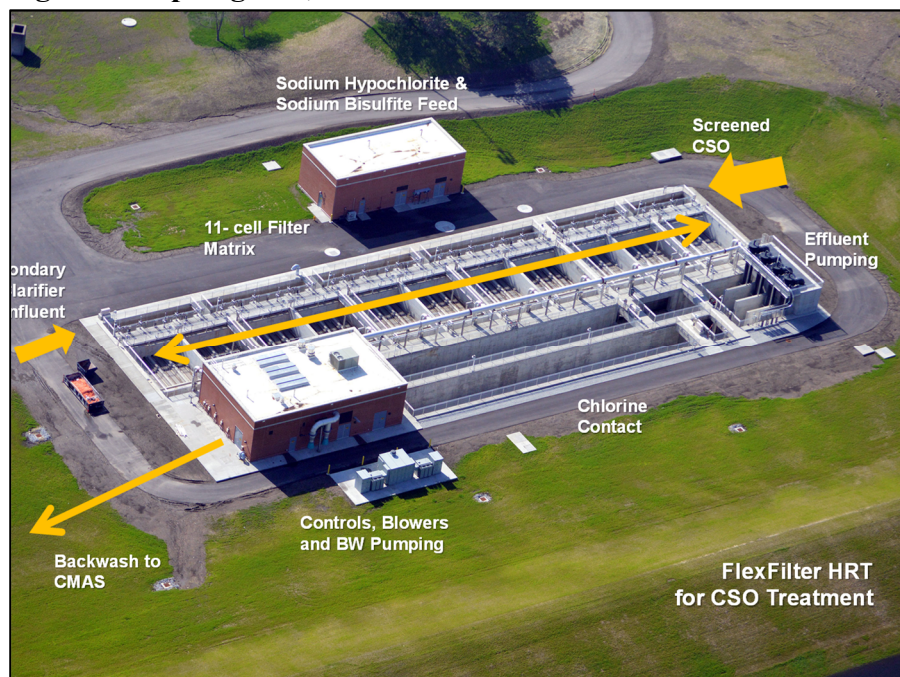
Figure 4 – Springfield, OH - FlexFilter EHRT Facilities
