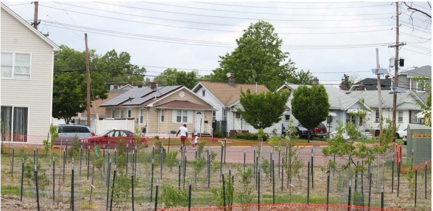
Post-demolition floodplain restoration on Blue Acres property in Linden, NJ.
